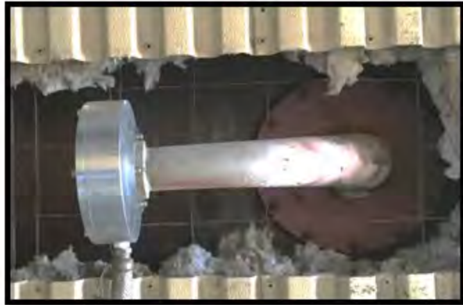
Picture 3 Lagging & Insulation Removed from Reactor Wall
