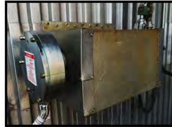
Picture 4 Insulation Box is installed around Bell Section B
