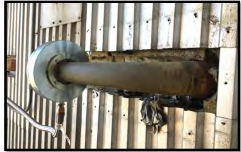
Picture 2 Bell Section A & Standard Sound Generator are replaced with the Magnum Sound Generator
