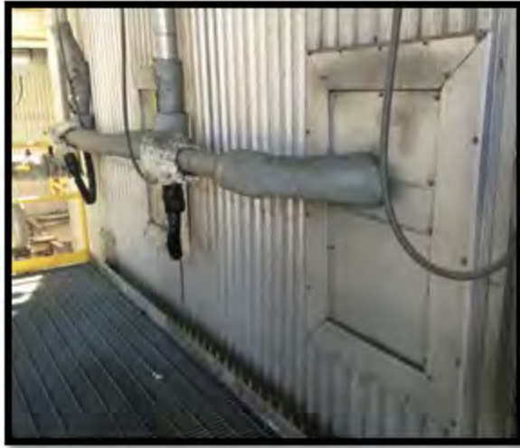
Picture 1 Model DC-75 Acoustic Cleaner Installation
